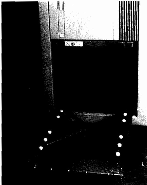
Figure 5-5. X-Brace Installed in Rack Slide
